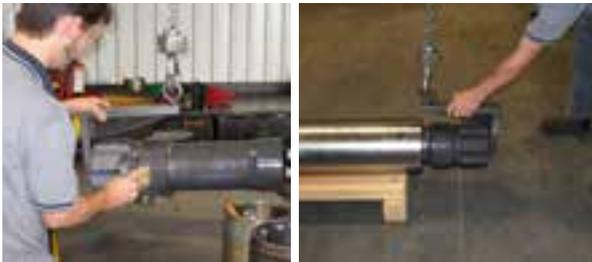
*Lubrication and installation of the piston.*
